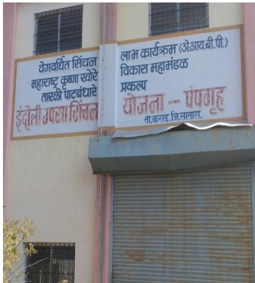
Fig 3.1 Pump House at Indoli
